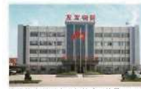
邯鄲基地-邯鄲友發鋼管公司外景 Appearance of Handan Youfa Steel Pipe Co., Ltd in Handan Base
