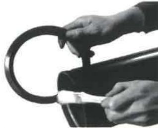
2. Lubricate gasket
