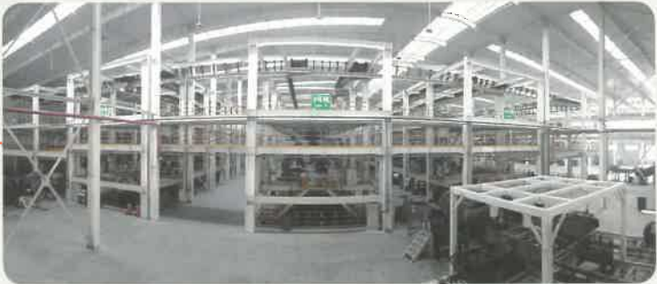
Threading, Air Pressure Test, and Anti-rust Treatment
