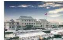
友發鋼管集團大樓外景 Appearance of Tianjin Youfa Steel Pipe Group
